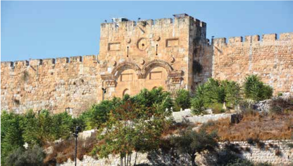
Golden Gate is the only eastern gate of the Temple Mount is 1 of only 2 that used to offer access into the city from that side. It has been walled up since medieval times
